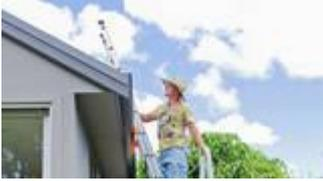
**Step 2:** When on a roof, you need to wear a harness connected to a securely anchored safety rope. Throw rope with at least 700kg breaking strain right over roof.
